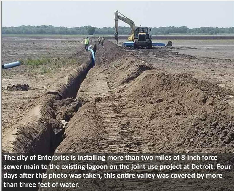
The city of Enterprise is installing more than two miles of 8-inch force sewer main to the existing lagoon on the joint use project at Detroit. Four days after this photo was taken, this entire valley was covered by more than three feet of water.
