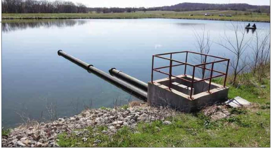
The discharge structure for this lagoon allows drawing effluent from two different depths of the final cell. Fortunately, the water level was down and the lagoon was not discharging so that this photo could be taken. Once a higher water level returns, the operator can then visually inspect water samples from each of the two depths to see which draw-off pipe produces an effluent with less green color and hopefully a lower Total Suspended Solids (TSS) concentration.
