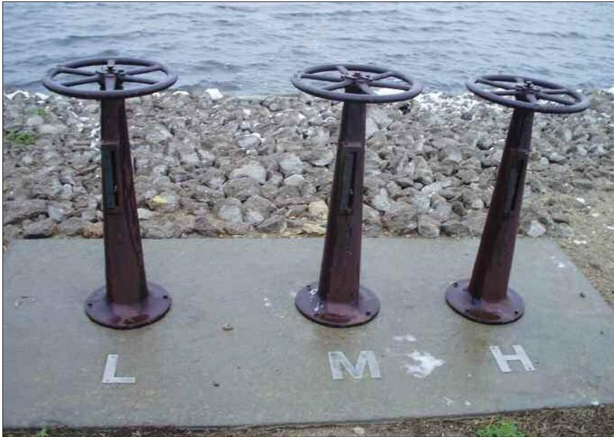
This lagoon is equipped with a discharge structure that allows drawing effluent at varying depths from the final cell. It is a good idea to "mark" each valve to ensure samples are collected properly. In this case, "L" is for the lowest draw-off pipe, "M" is for the middle pipe and "H" is for the upper pipe.
