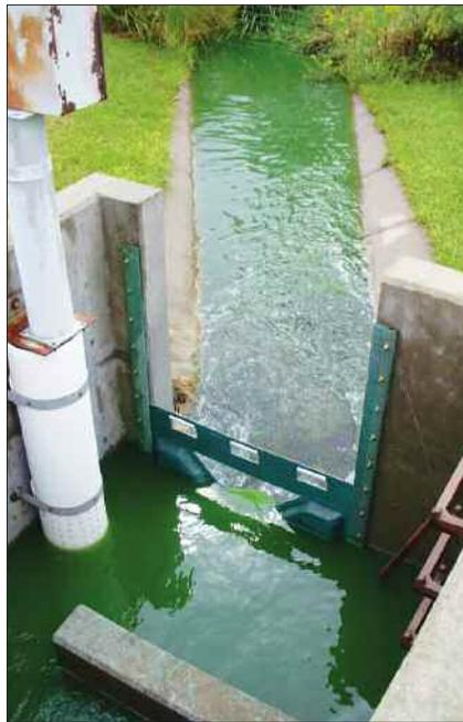
**This photo shows an example of a typical lagoon effluent during summer months. Notice the bright green color. The operator had sampled this effluent several days prior to the photo being taken. The TSS concentration was 96 mg/l which exceeds their limit of 80 mg/l.**
