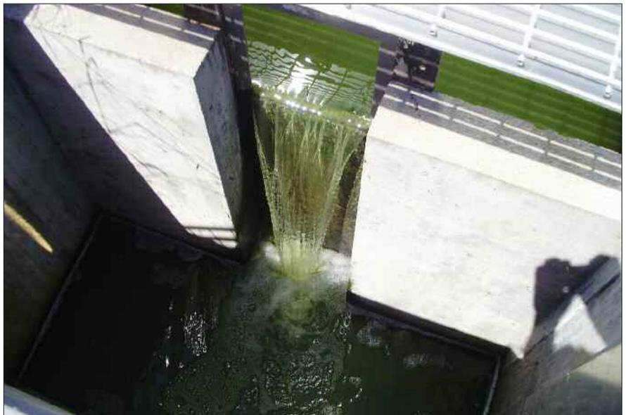
**This photo was taken during the summer and shows a lagoon producing a high-quality effluent low in Total Suspended Solids. If sampled, this effluent should meet TSS limits. Note that it has a slight green color, but not the concentrated green color found in the other photo accompanying this article. This lagoon happens to discharge off the surface of the final cell. But fortunately, sufficient algae die-off occurs prior to discharging.**
