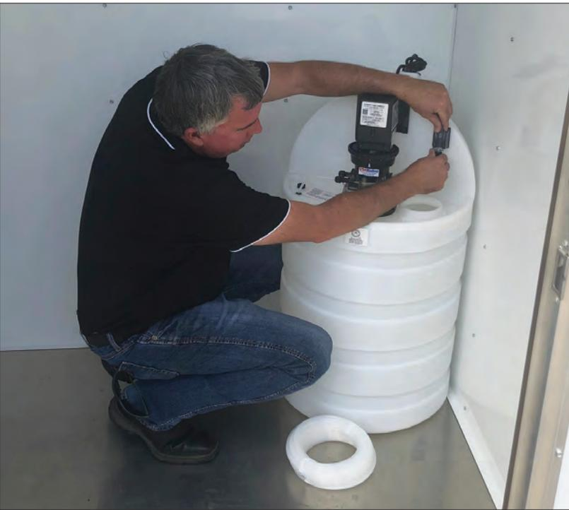
**Lonnie Boller installs a tank-mounted pump on the ammonia side of the rechlorination building**
