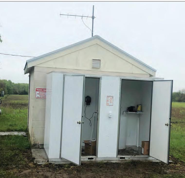
**This two compartment, portable rechlorination building was being placed at a booster station after a rain.**
