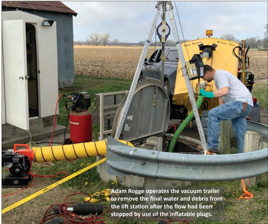
Adam Rogge operates the vacuum trailer to remove the final water and debris from the lift station after the flow had been stopped by use of the inflatable plugs.
