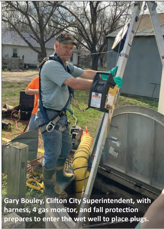
Gary Bouley, Clifton City Superintendent, with harness, 4 gas monitor, and fall protection prepares to enter the wet well to place plugs.
