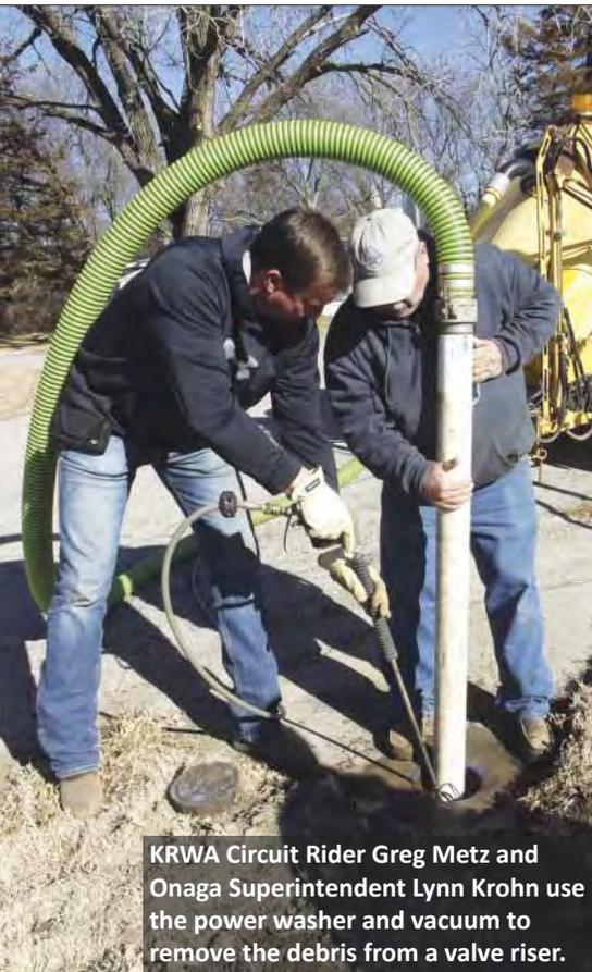
KRWA Circuit Rider Greg Metz and Onaga Superintendent Lynn Krohn use the power washer and vacuum to remove the debris from a valve riser.
