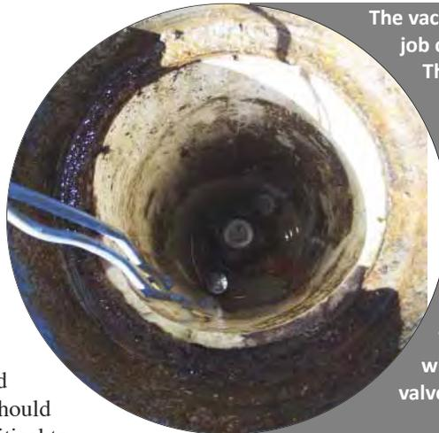
The vacuum does a very good job of removing debris. The valve can now be accessed. Note the locator wire does not go to the bottom of the riser. The wire was placed on the outside of the riser and then inserted near the top through a small hole. This protects the wire when operating the valve.
