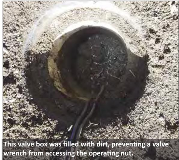
This valve box was filled with dirt, preventing a valve wrench from accessing the operating nut.
