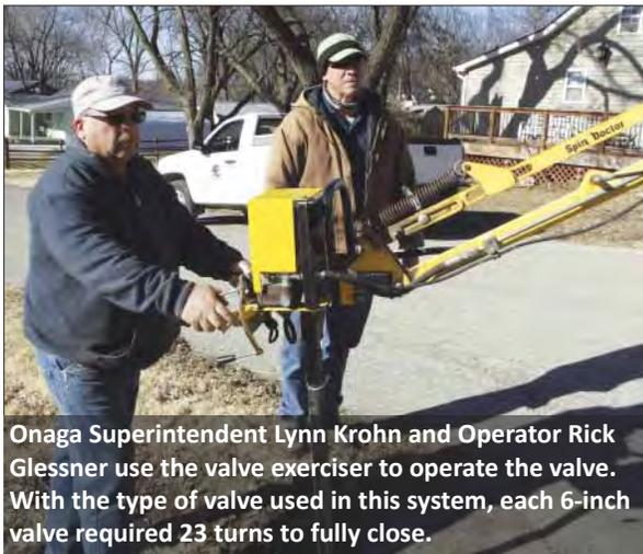
Onaga Superintendent Lynn Krohn and Operator Rick Glessner use the valve exerciser to operate the valve. With the type of valve used in this system, each 6-inch valve required 23 turns to fully close.
