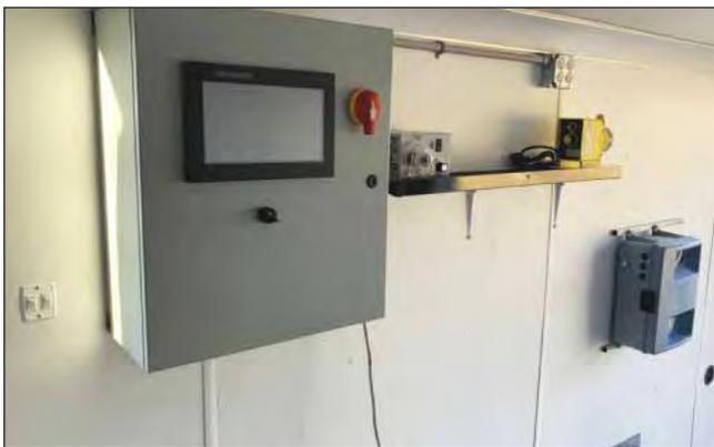
The training trailer will be equipped with a host of components used by water and wastewater systems. This photo shows a VFD and PLC which will control a pumping unit.
