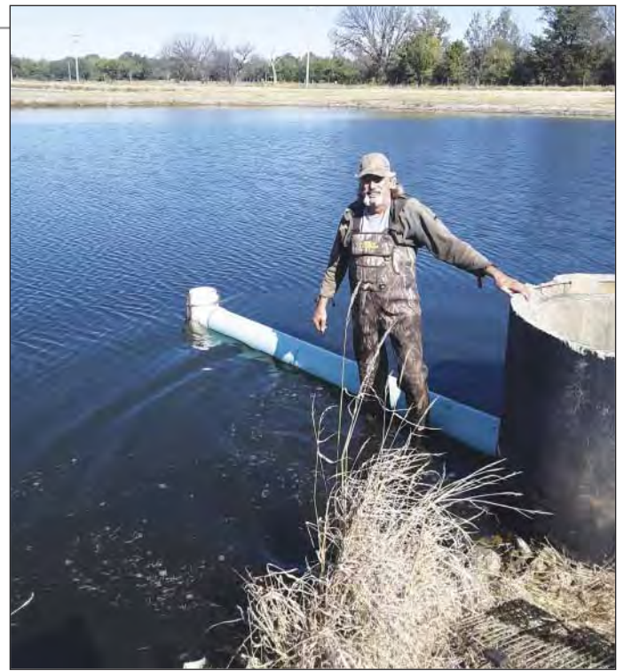
Rex Hess, city of Mound Valley Superintendent, is shown with the new pipe extension in place and operating. Since this improvement was made, the lagoon effluent's quality has improved and now meets limits for TSS and BOD.
