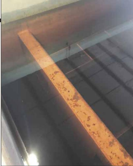
**Pink water on top of a filter, but was not dosed so high as to make it through the filter, which created ideal manganese results in the clearwell.**
