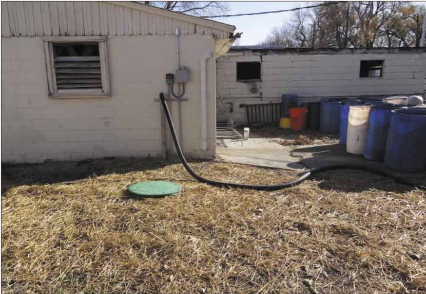
With the 1,000-gallon tank installed, note the black hose for pumping out the contents into the truck to haul it away. The electrical controls and high-water alarm are also mounted on the wall.
