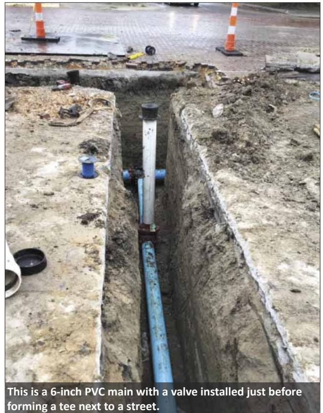
This is a 6-inch PVC main with a valve installed just before forming a tee next to a street.
