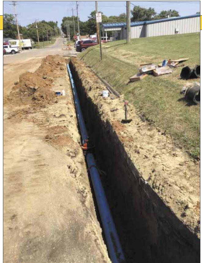
Shown here is an 8-inch PVC main recently installed on D Street on the south side of town, south of Highway 36.
