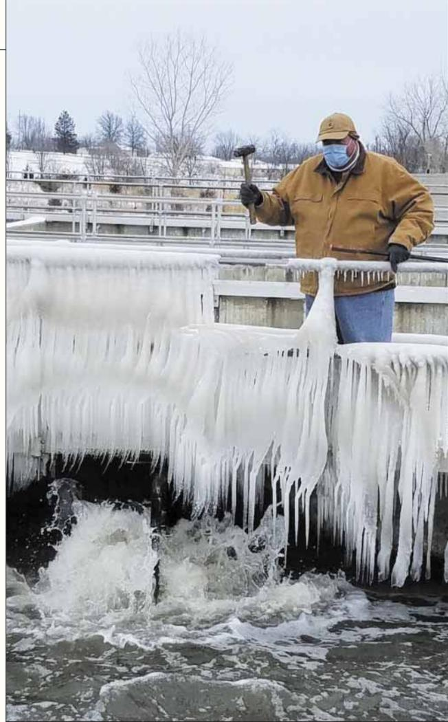
**City of Hiawatha Wastewater Superintendent Dave Grimm breaks ice off the railing near an air leak in the wastewater treatment facility in February 2021. The air leak caused the water to splash onto the rail and due to the extreme cold temperature caused ice formation.**
