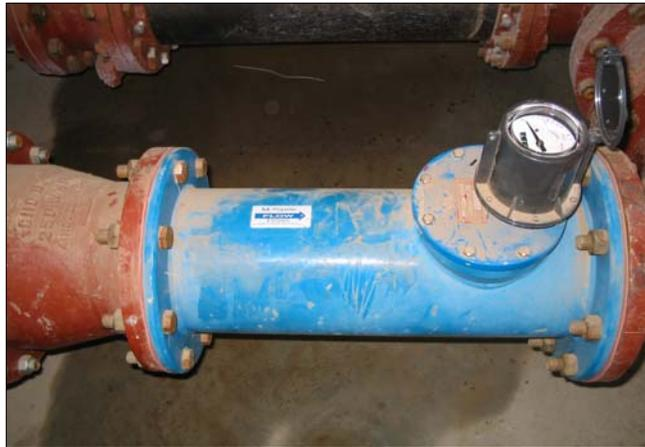
The above installation was made in 2003. This new meter is butted directly to reducers on either side.
