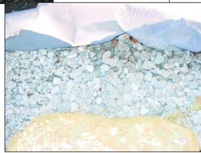
*This is a "Rock Bag" installed behind a limestone wall. The bag is used to alleviate the stress of excess moisture.*
