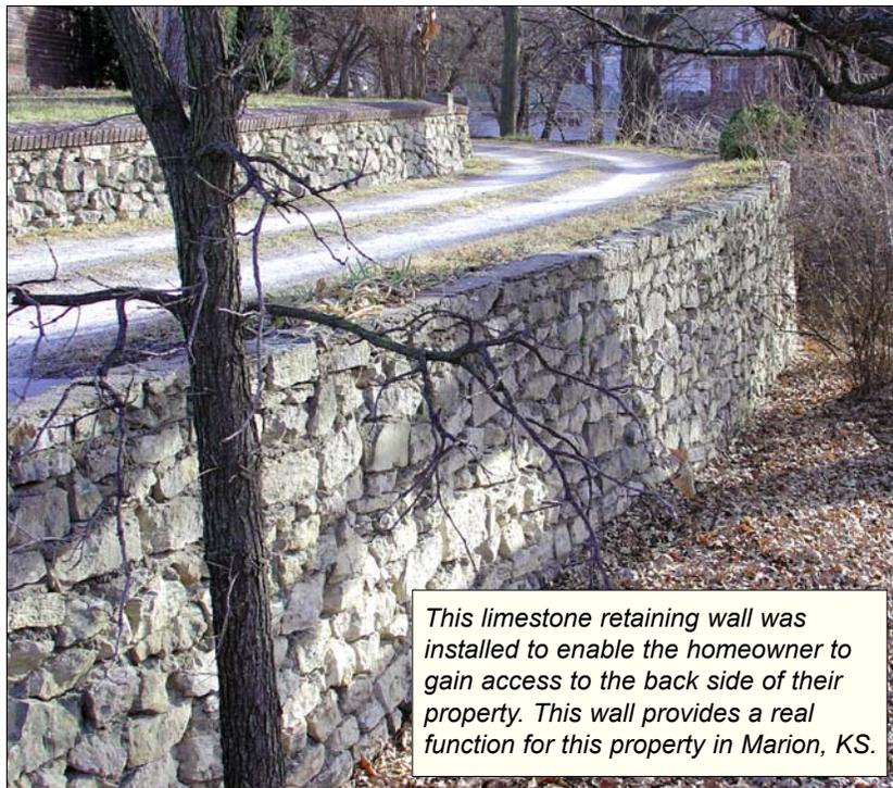
*This limestone retaining wall was installed to enable the homeowner to gain access to the back side of their property. This wall provides a real function for this property in Marion, KS.*
