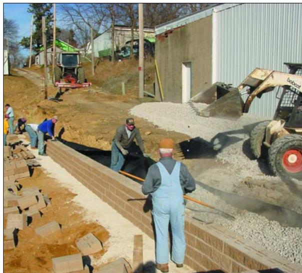
*This picture of KAN STEP volunteers at Goff shows backfilling with one-inch clean rock. The rock behind the wall will help provide adequate drainage and alleviate pressure from building along the backside. This wall runs from six and one-half feet down to three feet tall.*
