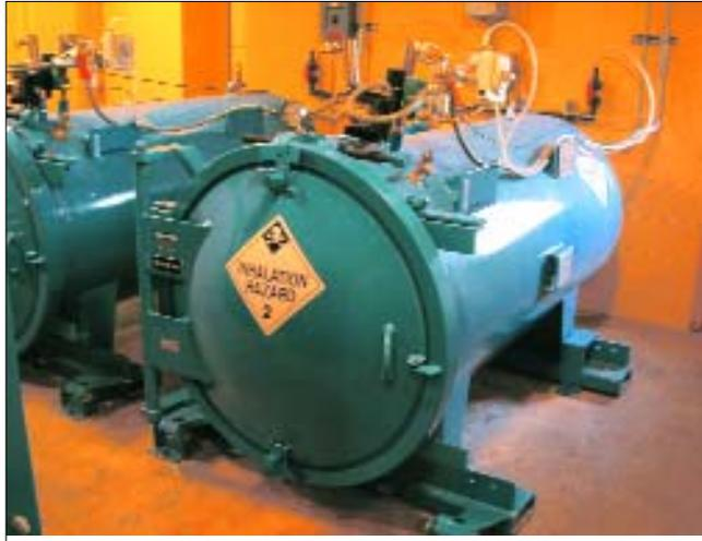
The above photo shows first of a kind chlorine containment equipment used in Kansas. These units each hold a ton chlorine cylinder. The units are part of the improvements being made by the Leavenworth Water Department.
