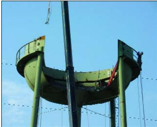
A close up of the tower tank shows the individual panels assembled by Caldwell Tank
