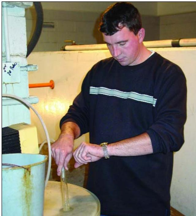
KRWA Tech Lonnie Boller is shown calibrating an ammonia feed pump at Valley Falls. The ratio of ammonia to chlorine is typically 3:1.
