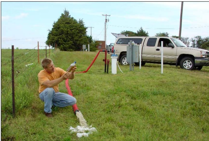
Steele shows a sample of the discolored water being pumped to waste during the treatment process. Treating well #4 improved specific capacity from 1.9 to 2.6. Specific capacity is a measuring expressed in gallons per minute per foot determined by dividing the yield by the drawdown.
