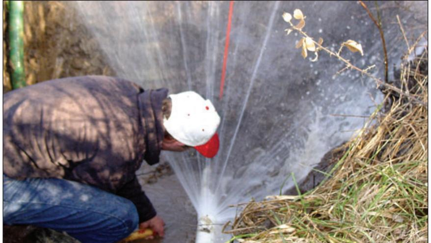
Willy Morrison, Crawford County RWD 4, works on a 50,000-gallon per day leak that required three weeks to locate. Found behind a brushy fence row and running away from the road ditch, this leak – like many others in RWDs – was difficult to locate. Once exposed and with valves that didn't fully close, this photo shows how an operator begins to make a repair.
