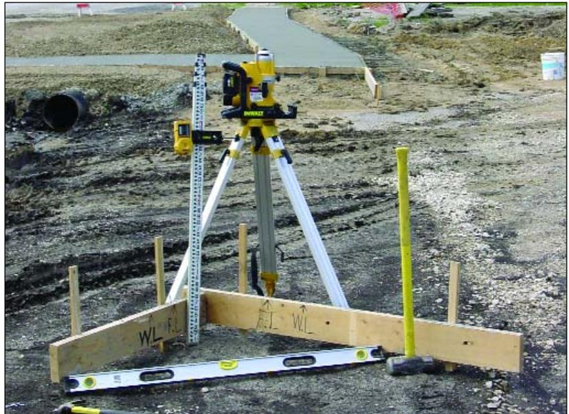
A set of batter boards is shown here marking a corner of the building layout. The laser transit seen in the picture helps locate the preliminary structures during this important first phase of construction. Note markings on batter boards, "WL" and "FL." Strings stretched from nails at these points will delineate the "wall line" and "floor line" of each of the building's elevations.
