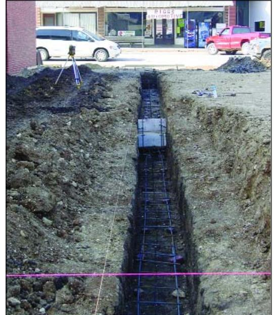
*The strings mark the building corner allowing footings to be formed “square” with adjacent structure and perpendicular to the road at top. Batter boards are seen at the top of the footing trench.*
