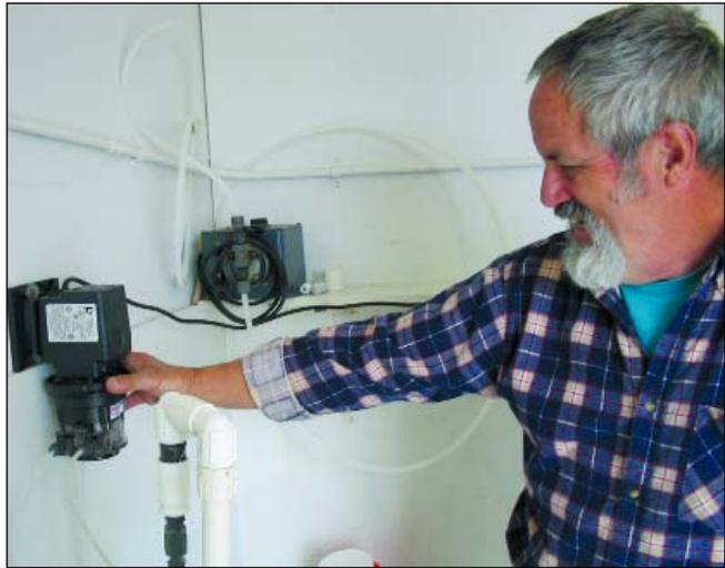
The city of Esbon's application of liquid chlorine solution has been trouble free since beginning use of the peristaltic pump. Operator Bob Windmuller is pictured above checking the unit.
