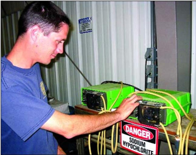
Gary Clark, operator at Mitchell County Rural Water District No. 2, checks adjustment on a peristaltic pump that supplies sodium hypochlorite to a contact basin in an effort to reduce TTHMs.
