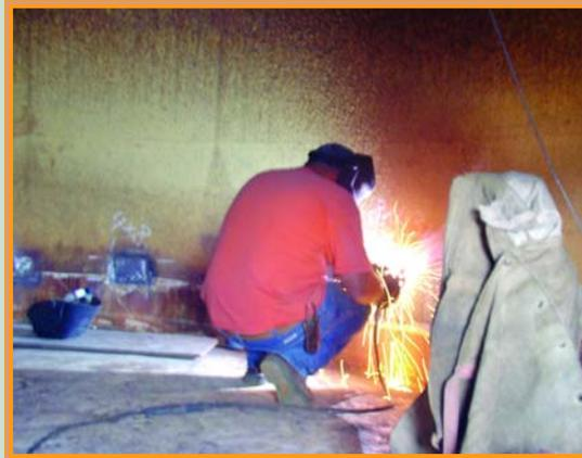
**Top:** Matfield Green Mayor Randy Talkington makes repairs to the city's water storage tank by welding steel plates over badly pitted areas.
