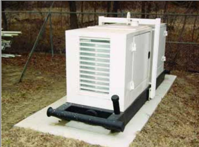
**Above:** This 50 KW portable generator was installed at Cherokee RWD 1 in 2005. The cost was approximately \$12,000
