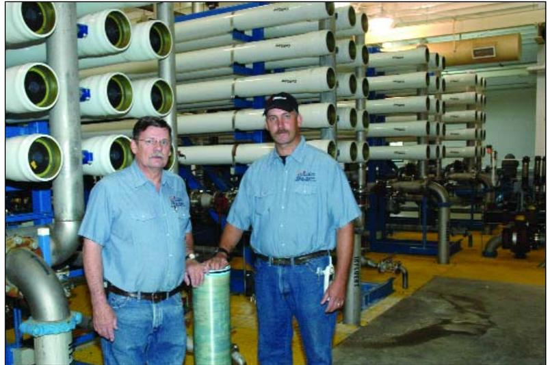
Norm Holt, water plant operator, and Jay Leusman, lead water plant operator, lean on a replacement RO membrane, 420 of which fit in the 60 tubes arrayed in the four skids behind them.
