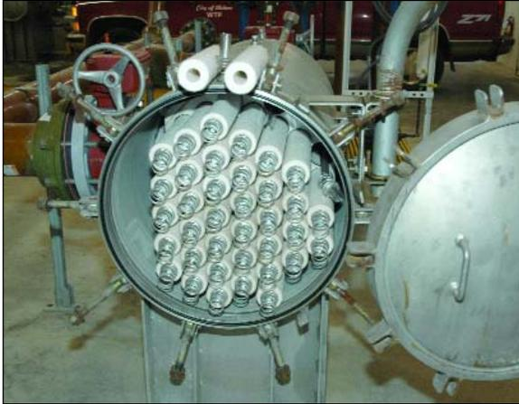
**Above:** Filter cartridges in the process are being replaced in the pressure cannister before water is pumped to the RO tubes.
