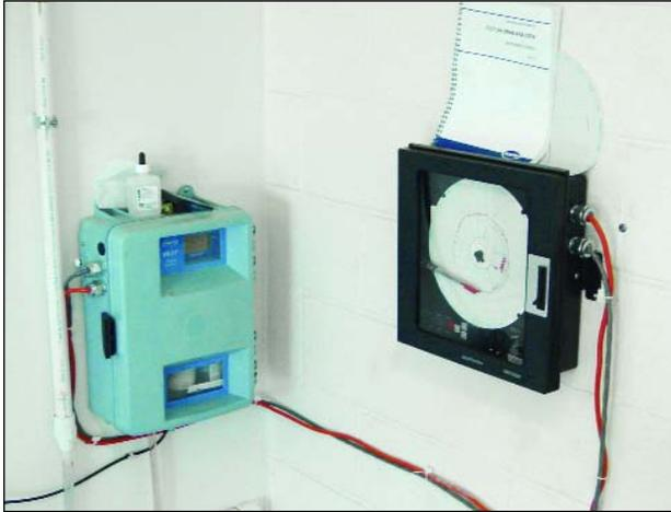
*When this chlorine monitor detects a chlorine residual of less than 2.0 mg/l, the feed pump turns on to add sodium hypochlorite to bring the residual up to 3.0 mg/l.*
