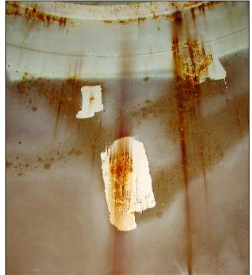
Another view inside the tank at Harper RWD 2. The lighter colored areas were recoated in a prior maintenance.
