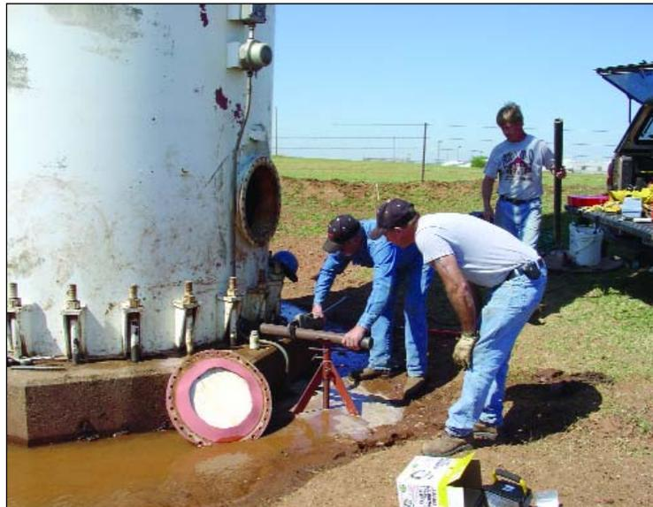
Rick Harnden and Ron Kasal, members of the board of directors at Harper RWD 2, use a special tool that KRWA Tech Jon Steele, standing behind, provided to remove the drain plug on this standpipe.
