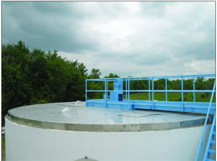
*The Pleasanton water plant clarifiers have new stainless steel covers. One is seen on the clarifier shown above. Part of the new catwalk between the two clarifiers is also shown.*
