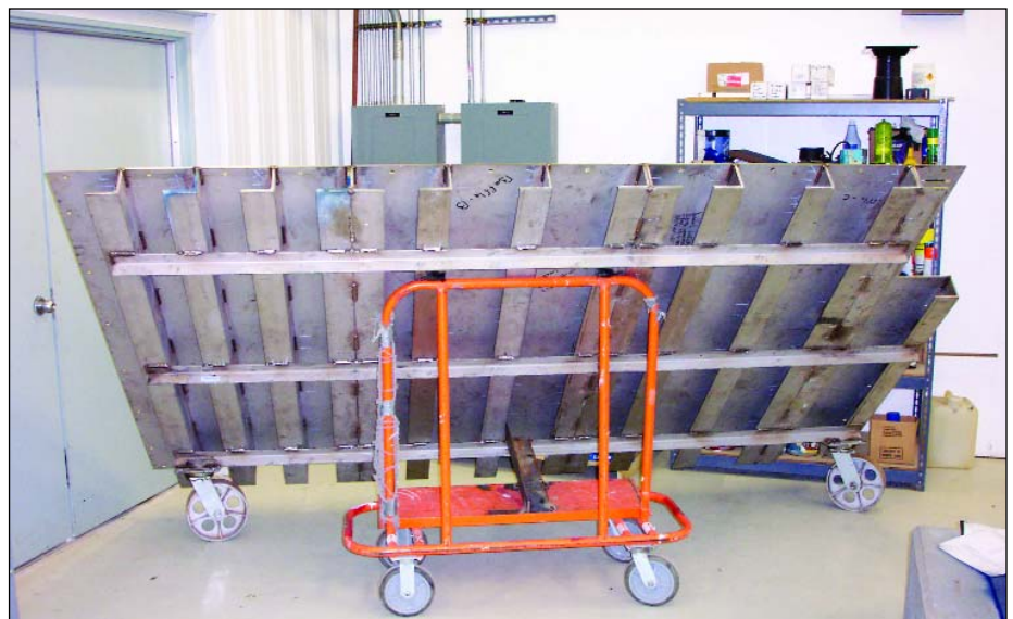
The divider/overflow wall constructed of ¼-inch stainless steel plate and stainless angle irons on a cart before installation. Because of the 1,800 pound weight, temporary wheels were welded to the downside corners of the wall construction, carrying some of the weight.
