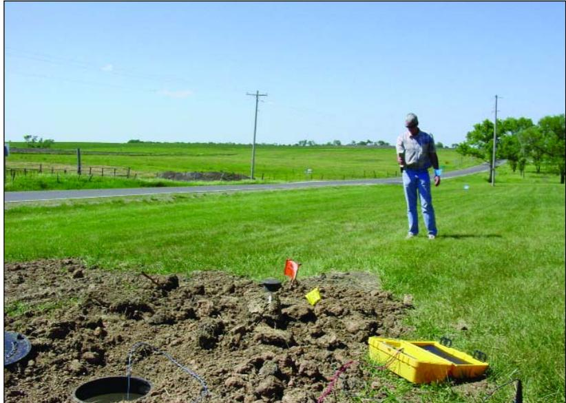
*Using an electronic locating device, as demonstrated by Nemaha RWD 3 Manager Paul Strathman, may be more reliable assuming the tracer wire hasn't been cut or stripped during installation.*
