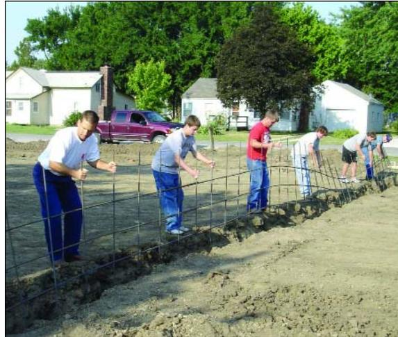
**Above left:** The Uniontown High School Trades Class sets the floor drain trough before the concrete slab floor is poured.
