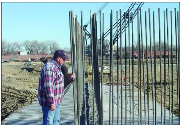
Sewer Plant Operator G.D. Hite stands on the three foot thick footings for the basin walls. Rebar is in place ready for forms to be set so the basin walls can be poured.
