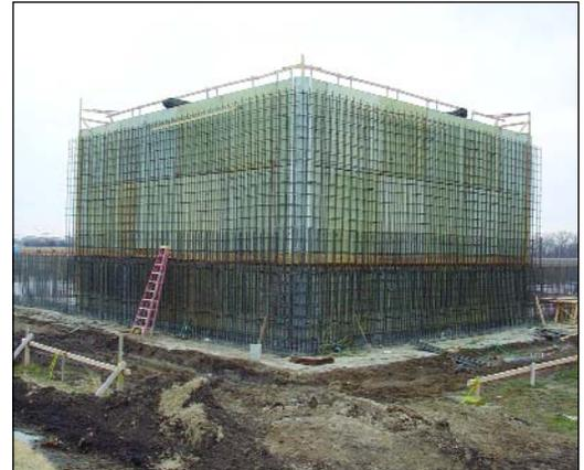
The new plant basin is under construction. Inside forms are in place with wall strengthening steel being tied-in before the outside forms are set.
