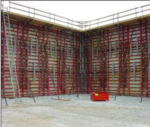
From inside the plant basin, form sets and bracing pieces are seen being readied for pouring the 25 ft. tall concrete walls.
