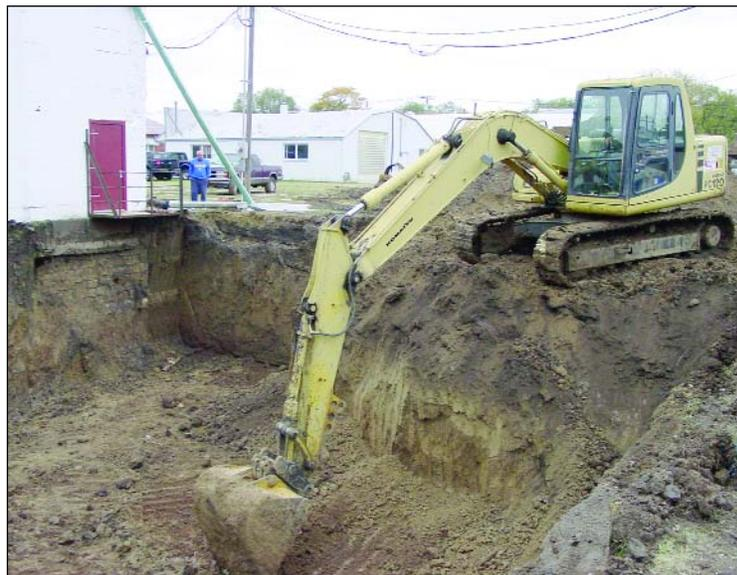
*The photo shows excavation that is nearly finished, with the operator pulling earth from the last corner of the addition's basement. Over 1,000 cubic yards were removed for the project. A skid steer loader was later lowered into the hole to smooth and level the floor before construction of footing forms.*
