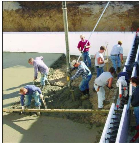
**Center:** The concrete pumper truck is giving the basement floor volunteer crew all they can handle but they won't be finished until they fill the first section of foam ICF wall forms around the perimeter of the floor.
