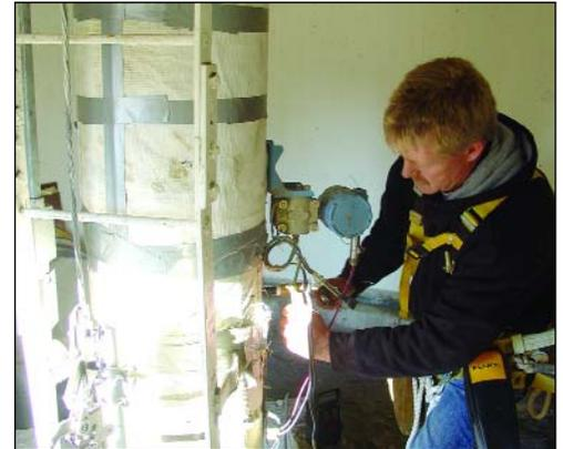
**Right:** Jon Steele puts finishing touches on the fitting welded to replace the one that ruptured.
