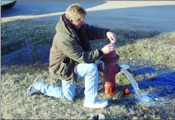
**Above:** To make sure it is safe to get the tank back on line, Jon Steele caps a sample bottle to submit to a lab for a test of bacteriological quality. This hydrant is at the base of the tank and is regularly used as the sample site.
