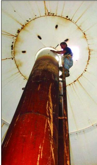
**Center:** Jon Steele inspects the riser top that will be extended to top of the tank where a new hatch will be built. This will change the riser pipe exit route to the tank's exterior.
