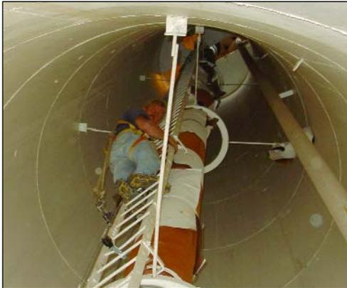
**Above:** Jon Steele, in his safety harness, inspects vendor's work on pipe insulation and ladder bracing.
