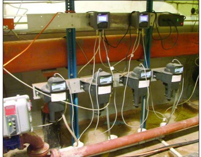
*Pictured above is a view of online turbidity monitoring equipment installed as part of the 2000 upgrade project.*
