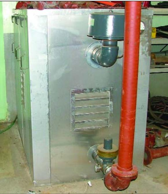
The blower unit above was installed to operate the air scourer system at the filters.
