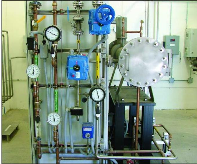
**Left:** The machine pictured is one of two Mitsubishi ozone generators in use at the water plant.
