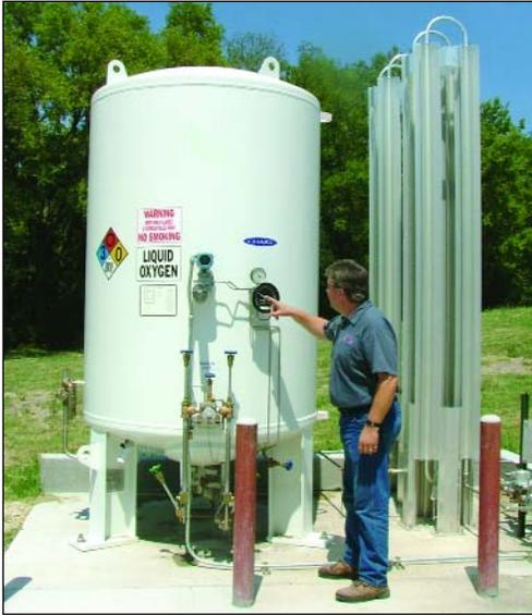
**Far Left:** Operator Marty Fredrickson checks a control on the plant's liquid oxygen storage tank. Ozone is generated from the liquid oxygen.
