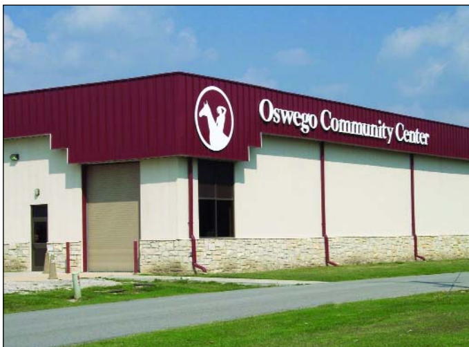
The new community center in Oswego was also constructed using grant funds from a comprehensive development grant. The new community center is a focal point and is used for family reunions, fair exhibits, civic groups and recently a music festival.
