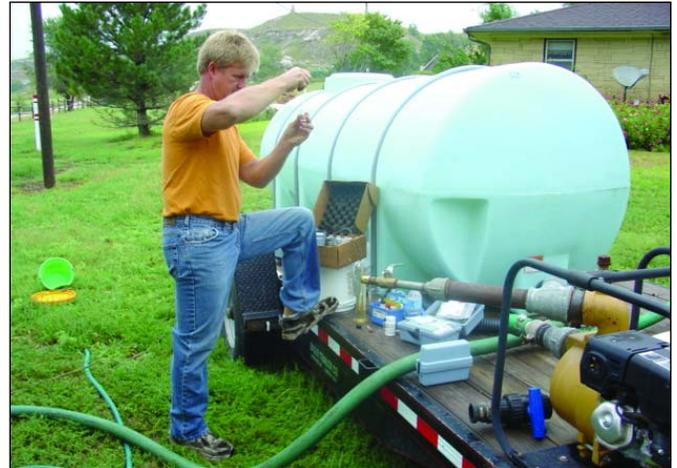
KRWA Tech Jon Steele is shown checking water chemistry after the treatment solution was introduced and surged in the well.
