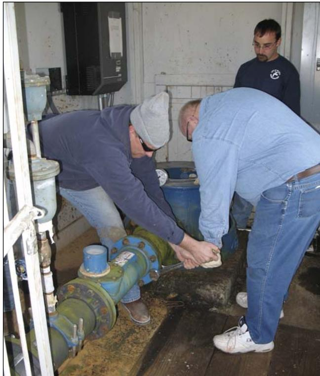
*Top: This image shows one of the new water meters that was installed at the city wellfield. The new master meters helped to correct the city's 'unaccounted for' water losses by more than 350 gpm.*
