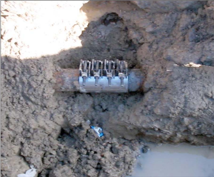
Doug Guenther affixed the full circle leak repair shown above. Because of the wind and cold weather, the city repair crew was happy to see the leak's excavation backfilled and the patch put on the highway surface above.
