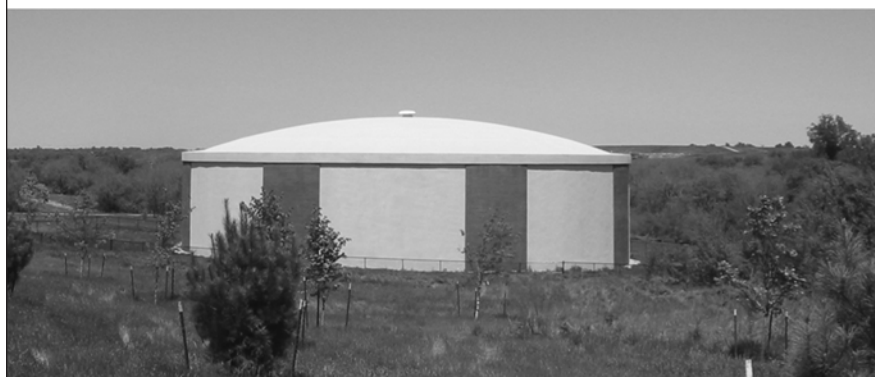
6.0 MG Natgun water storage tank for the City of Olathe, KS. Engineering by Burns & McDonnell Engineering Co.
