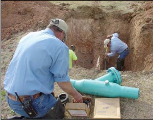
Doug Graff (kneeling) and Richard Foster prepare the launcher and valve to be installed in the force main.
