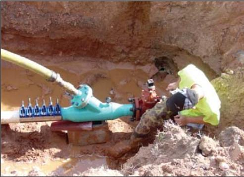
Preston Trotter of Mayer Specialties checks the pressure gauge used in determining if the line has been cleaned.
