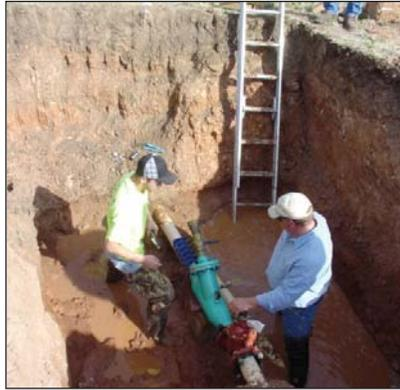
The pig launcher is installed with a valve to allow inserting the pig into the main without having backsiphonage of wastewater into the pit each time a pig is needed.
