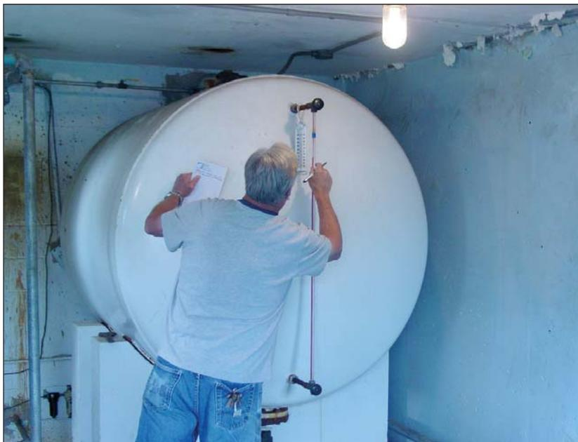
J.W. Stephenson, operator at Cherokee RWD 2 at Riverton, Kan., checks pressure and water levels in one of the district's hydro-pneumatic tanks. This design concept was used extensively on water systems constructed in southeast Kansas.
