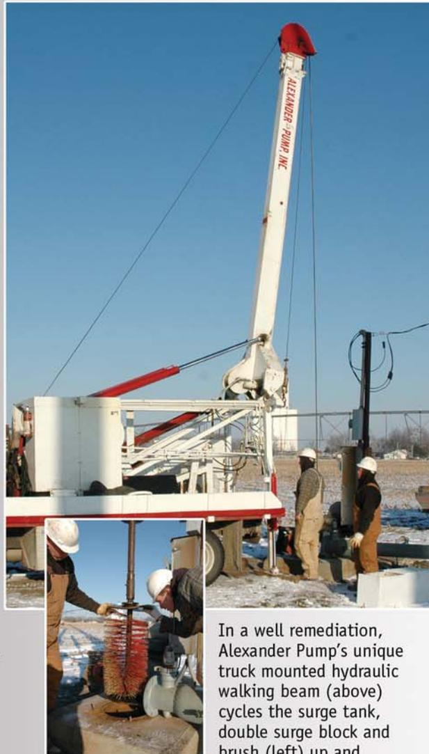
In a well remediation, Alexander Pump's unique truck mounted hydraulic walking beam (above) cycles the surge tank, double surge block and brush (left) up and down through the well. The action forces 'Redi Clean' chemicals into the gravel pack to dissolve iron bacteria, placing it into suspension for removal.
