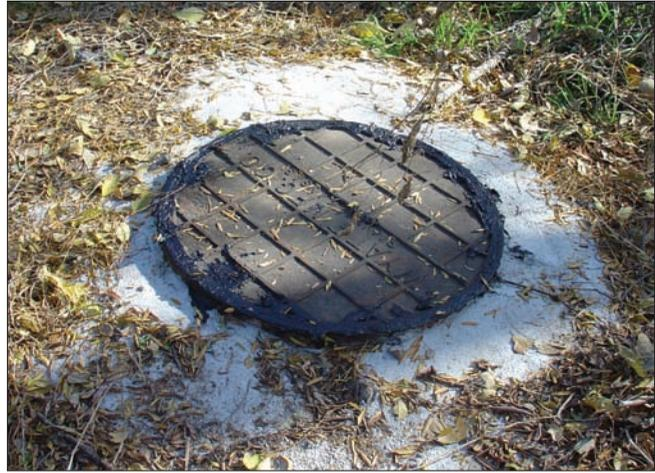
**This manhole is located in a low-lying area. It was raised and sealed to prevent inflow.**
