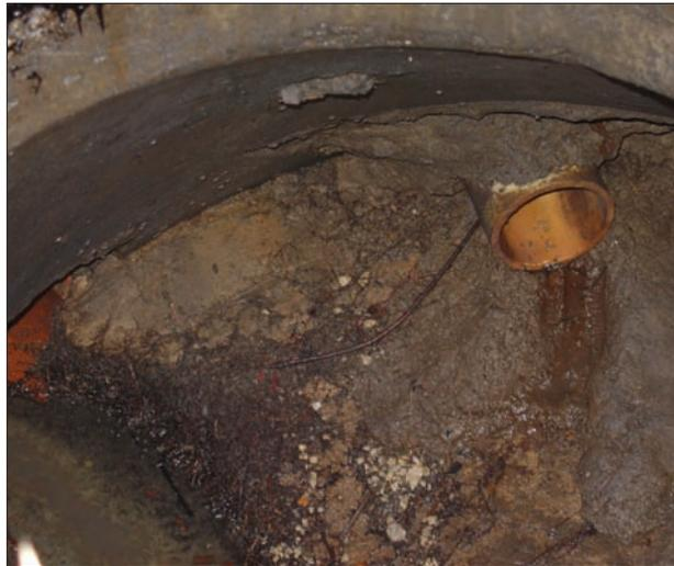
This photo shows a 4-inch service line that had serviced a trailer court which has not had a trailer for more than 10 years. But note the obvious flow line inside that pipe. The uncapped service connection in the trailer court were adding much additional rainwater to the collection system.
