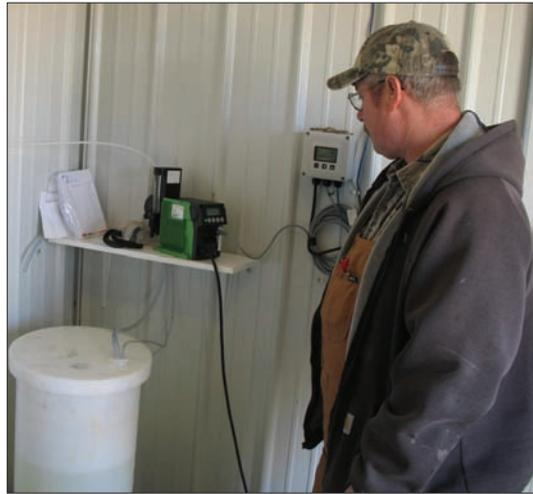
**Steve Geiger, Water Operator for the city of Uniontown, checks the pump at the rechlorination station that belongs to Bourbon County Consolidated RWD 2. The city of Uniontown purchases all of its water from Bourbon Cons. 2. This station has helped the city to maintain its chlorine residuals.**
