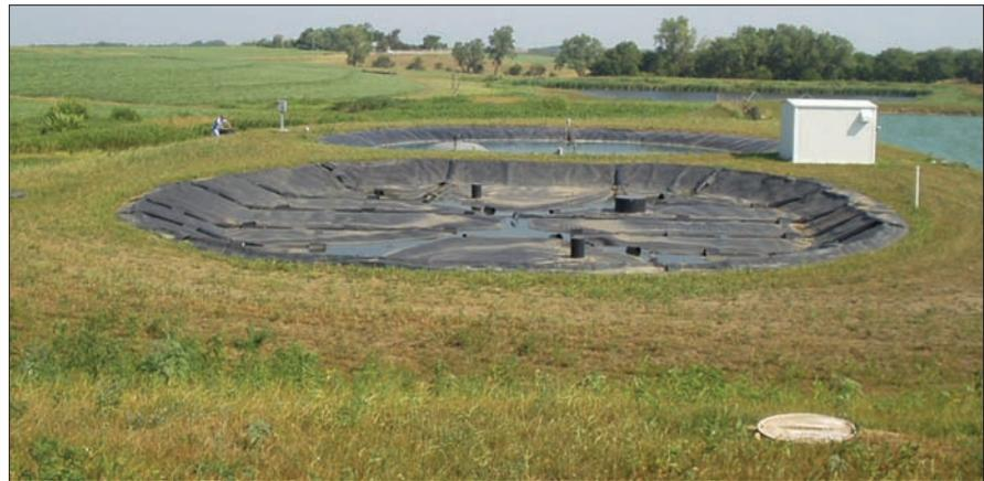
The city of Bern’s three-cell lagoon receives wastewater from a local dog food manufacturer after pretreatment. The pretreatment system consists of a covered anaerobic basin followed by a mixed, aerobic basin and settling basin. Sludge must be periodically removed from the anaerobic basin and disposed of properly. In the past, the city has land applied the sludge.
