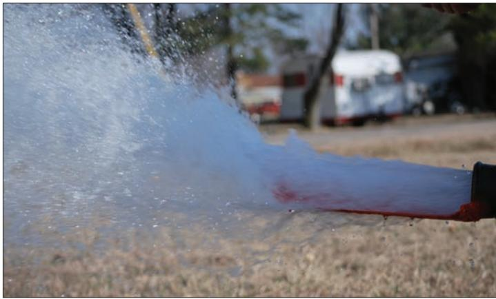
**It is generally accepted that a velocity of about 2.5 to 3 feet per second (F.P.S.) will begin moving sediment in piping.**
