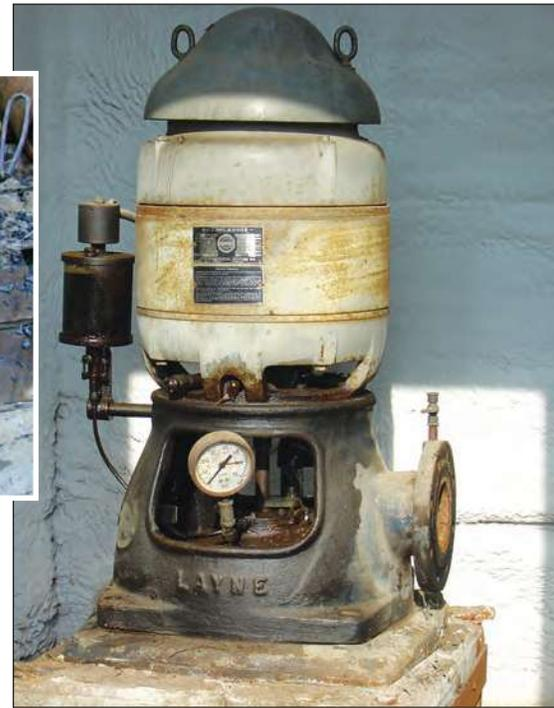
This 10-HP 3-phase motor operated the well that provided supplemental fire supply water to the town of Morrill.
