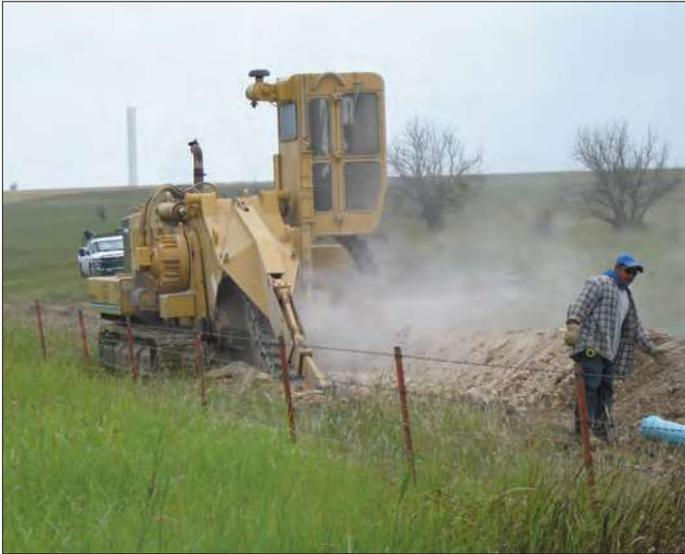
**Creating a little dust as it cuts its way through some rock, this 1455 Vermeer trencher has little trouble cutting through. PWWSD 20 is adding new 8-inch, 6-inch and some 4-inch PVC lines; Nowak Construction Company, Inc. of Goddard, Kansas is the contractor for the pipeline**
