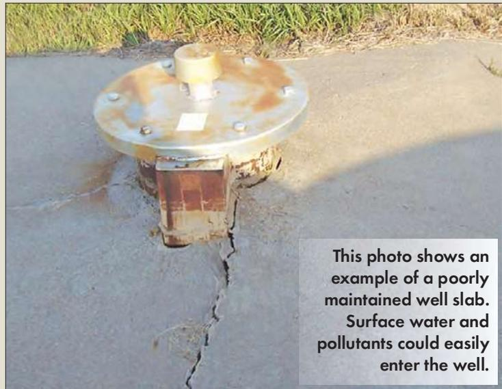
This photo shows an example of a poorly maintained well slab. Surface water and pollutants could easily enter the well.
