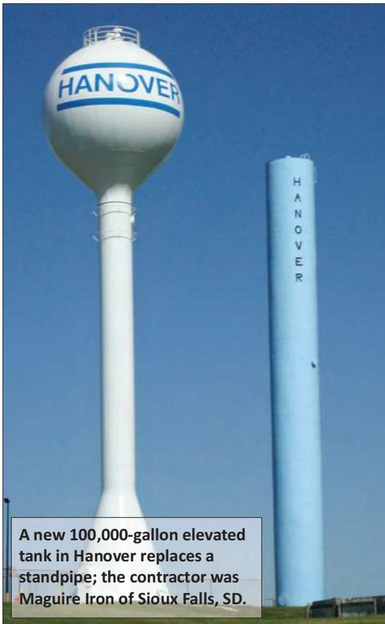
**A new 100,000-gallon elevated tank in Hanover replaces a standpipe; the contractor was Maguire Iron of Sioux Falls, SD.**
