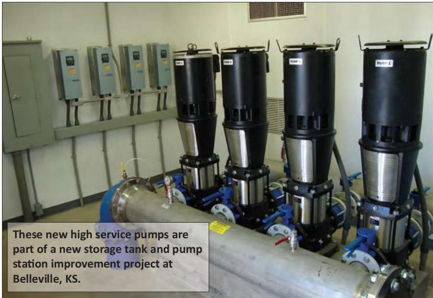
These new high service pumps are part of a new storage tank and pump station improvement project at Belleville, KS.
